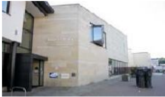
Durham City Customer Access Point
