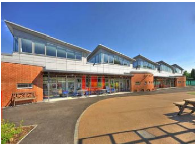
Brandon Primary School – New Build
