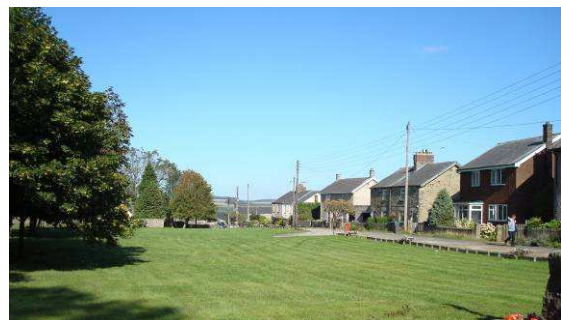
The properties of Hall Road differ in age and design, but are unified in their orientation to the street, their 2 storey height, and the arrangement of space around them.
