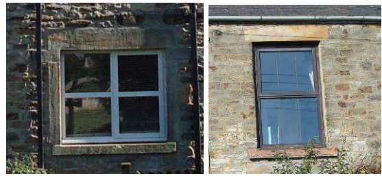
Openings of buildings of Esh have stone lintels and cills
