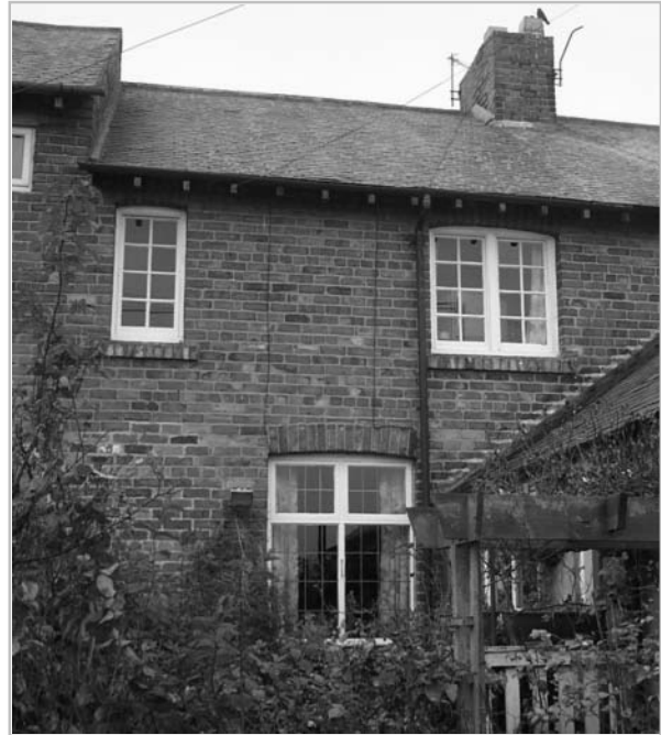
7 – Original fenestration to upper floors, UPVC replacement on the ground floor.
