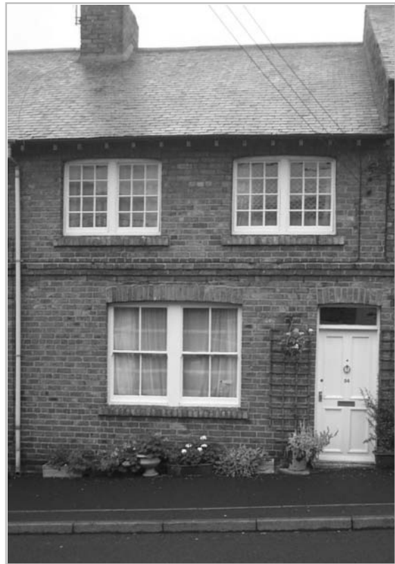
3 – Number 54 Stevenson Street, well preserved original features.
