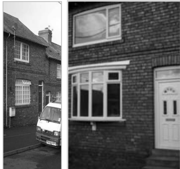
6 – Above, loss of chimney pots, prominent meter box and satellite dish, replacement UPVC windows and doors.
