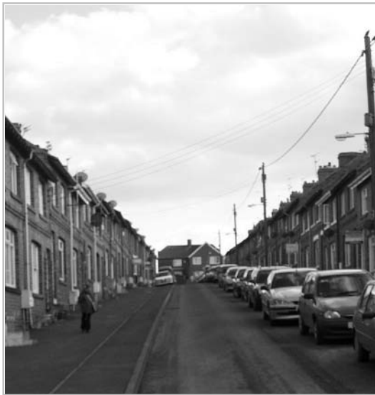
2 – The view north – south up Stevenson Street, the original built form still very evident today.
