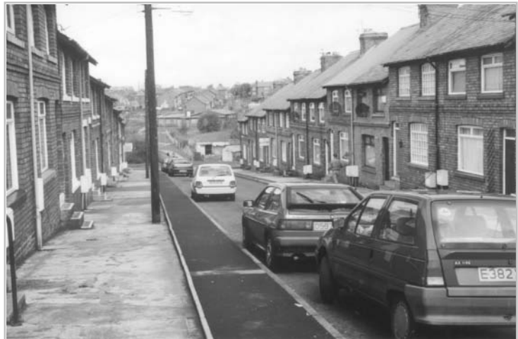
Above – satellite dishes on the street frontage, UPVC windows, prominent gas metre boxes and plastic rainwater goods.
