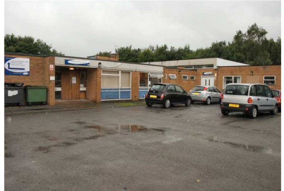
Car Park and entrance to the Lighthouse Resource Centre
