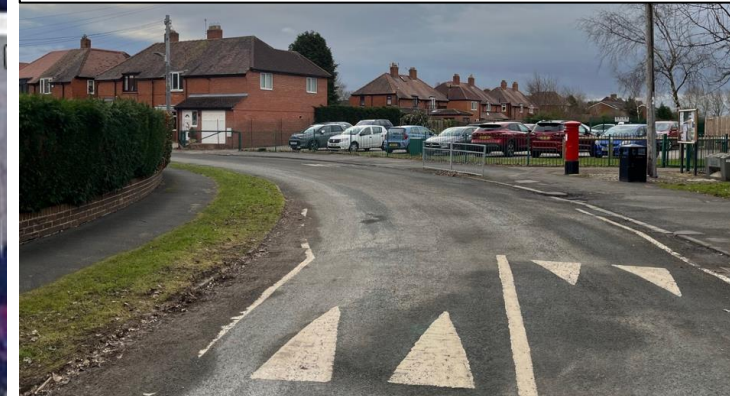
Visibility of approaching road users is restricted by the nature of the carriageway.
