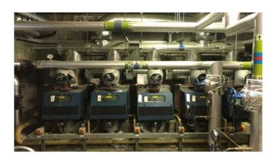
The boilers in a poor condition for their age and in need of replacement.
