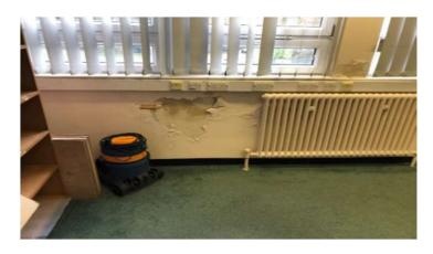
Internal Walls within medical records area in poor condition large areas of damp, staining and plaster damage.
