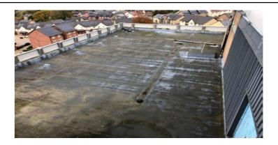
Flat Roof above the medical records to the lower ground floor, causing damp internally.
