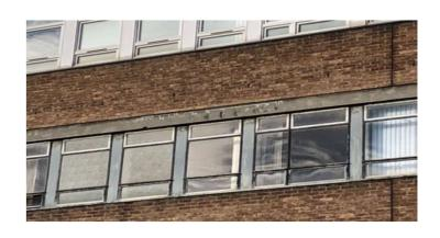
External Elevation - Horizontal concrete banding visible in poor condition
