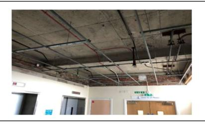
Suspended ceiling exposed as part of ACM removal works suspended ceilings have reached end of useful life.
