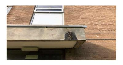
External The concrete canopy is in poor condition with localised spalling
