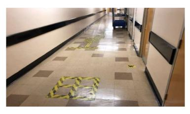
Floor Finishes Vinyl floors in poor condition heavy areas of straining and missing floor tiles
