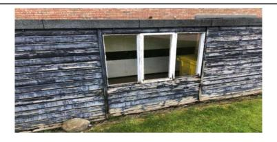
External Timber shiplap cladding is in a very poor condition and in a dilapidated state. There are several areas of timber decay visible to cladding
