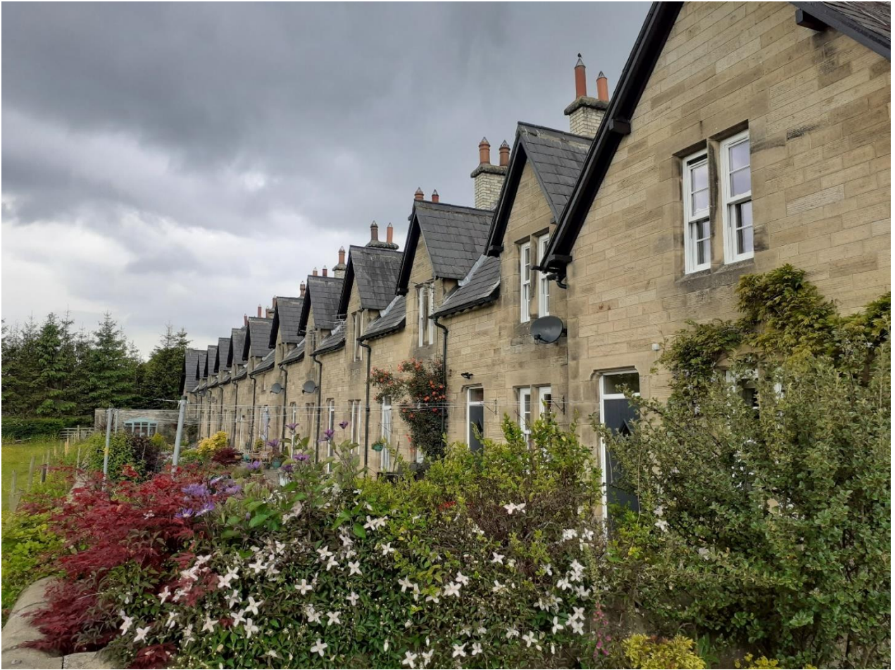
Terrace of 12 Almshouses built in 1860-1, Staindrop. An example of an asset identified on a Local List.
