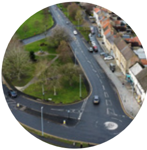
3,845 km of highways
