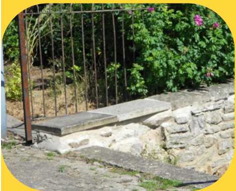
The wall after repairs.
