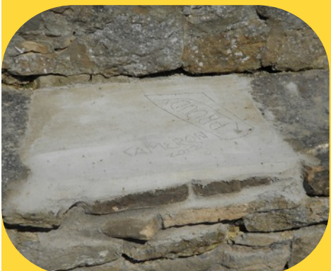
The seat after it had been repaired.
