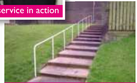
New handrail at Oakerside Drive
