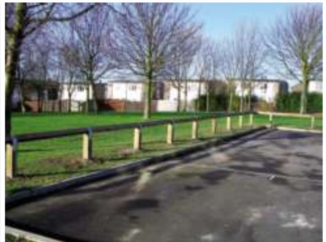
New fencing at Hovingham Close car park
