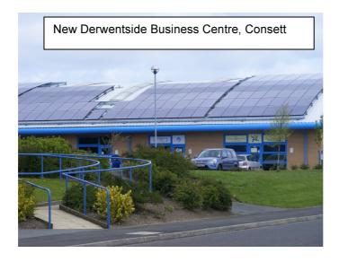
The panels should generate over 707,000 kilo watt hrs annually in free electricity, around £230,000 income per annum from the Government Feed in Tariff Scheme and save 350 tonnes each year in carbon emissions. The total cost of the project
