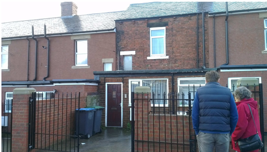
Improved/Non-Improved Group Repair Properties at Craghead
