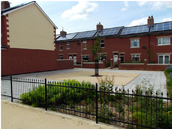
Environmental Improvements and Solar Panels in Craghead
